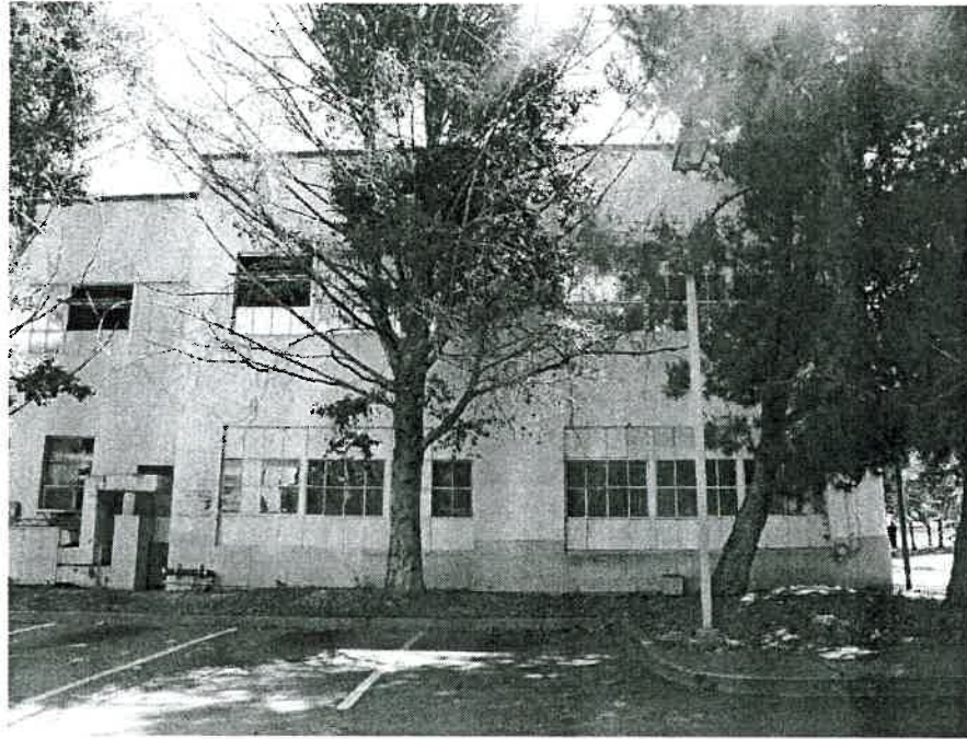
Figure 11: South end of southwestern elevation of 1928 portion of Building 800. (Carey & Co. Inc., 2006)
