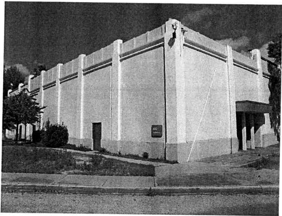
Figure 10: The northeast and southeast elevations of the 1928 portion of Building 800. (Carey & Co. Inc., 2006)
