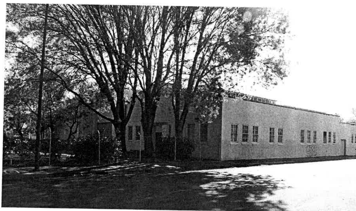
Figure 6: February 2008 view of northeast and northwest elevations of c. 1919 portion of Building 800. (Carey & Co., Inc.)
