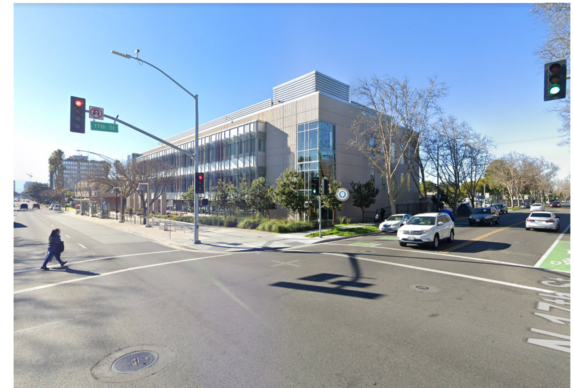
VIEW FROM EAST SANTA CLARA ST. & N. 17TH ST. 1
